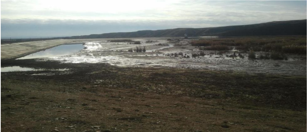
Fig.1: Pirsatchay water reservoir built in 1964 with a total area of 16.9 million m 3 (2017)
